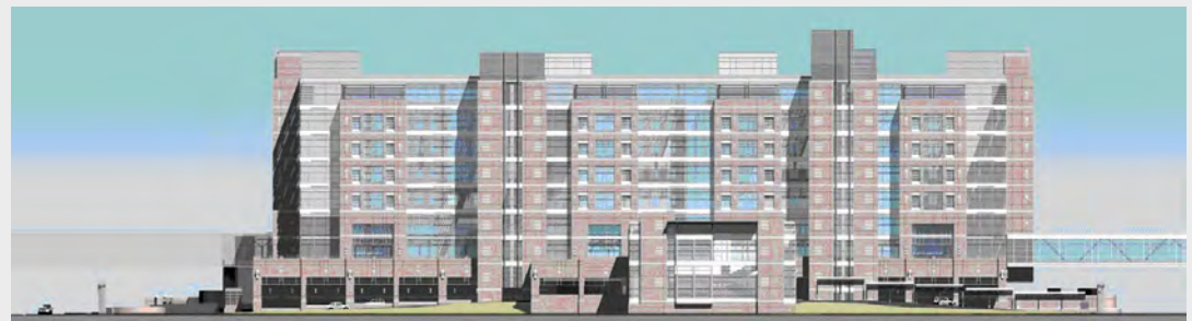
University of Texas M.D. Anderson Ambulatory Care Facility
