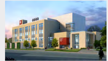
University of Houston Multi Disciplinary Research and Engineering Building
