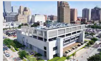
Union Station Central Energy Facility
