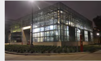
University of Houston Central Plant Upgrade
